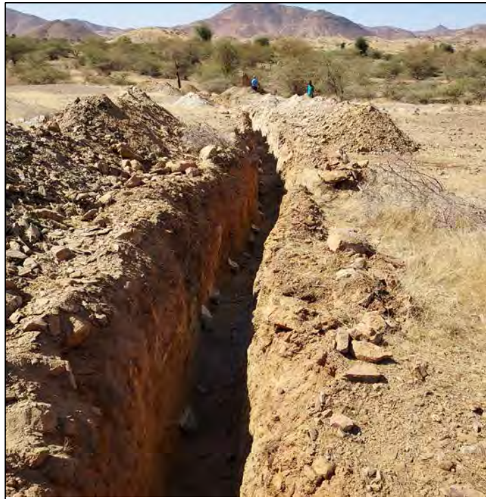
Trenching programme at Kerkasha
