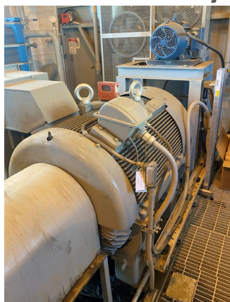
Bantry 2-29 600 hp Compressor recently replaced
