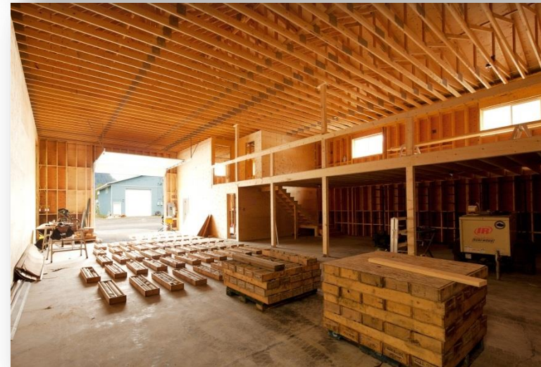
Stewart warehouse constructed by development corporation of Skii km Lax Ha First Nation
